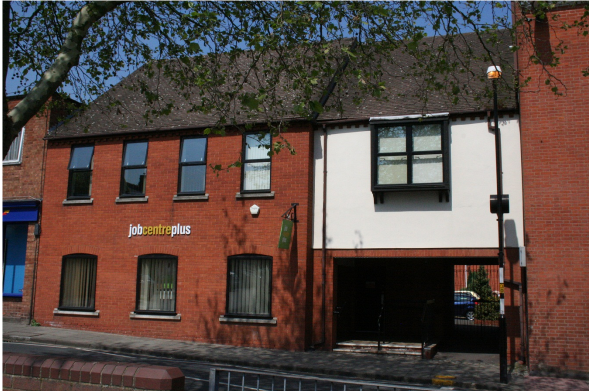
Front view of 120 Long Street – from Public Car Park in Long Street/Woolpack Way
